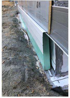
Figure 5: Slab Edge insulation with flashing and protection.
