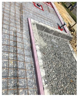
Figure 4: Stem Wall insulated to height of Slab. Insulation to be cut at 45 degree angle away from wall (2018 VRC Code Section N1102.2.10 (R402.2.10))
