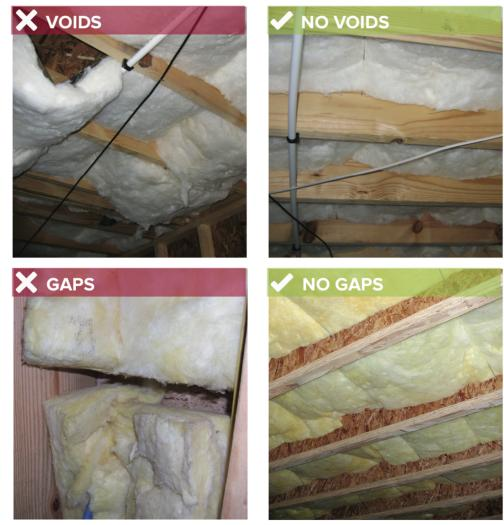
**Best Practice:** Cut and split insulation around all blocking, plumbing, HVAC, and electrical components to obtain a completely full framing cavity.
