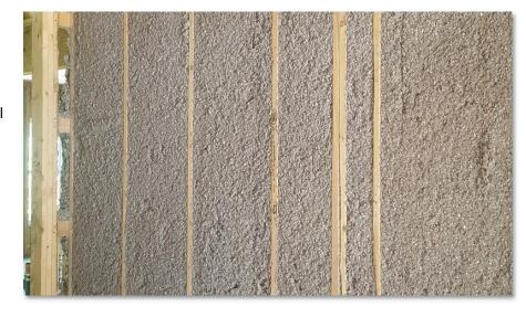
Figure 3: Damp-spray cellulose insulation in wall
