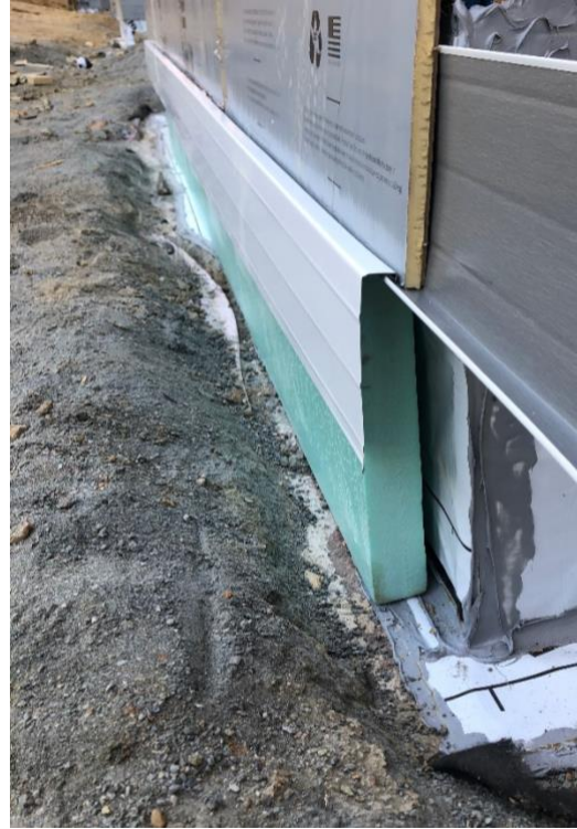
Figure 5: Slab Edge insulation with flashing and protection.
