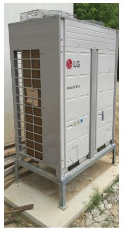
Figure 4: VRF outdoor unit is set on a pad on the perimeter of the building.
