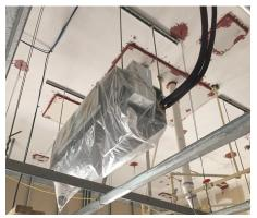
Figure 2: Diligent ceiling unit airsealing by KBS improved the compartmentalization and overall airtightness of each apartment, reducing energy consumption, and improving indoor environmental quality.
